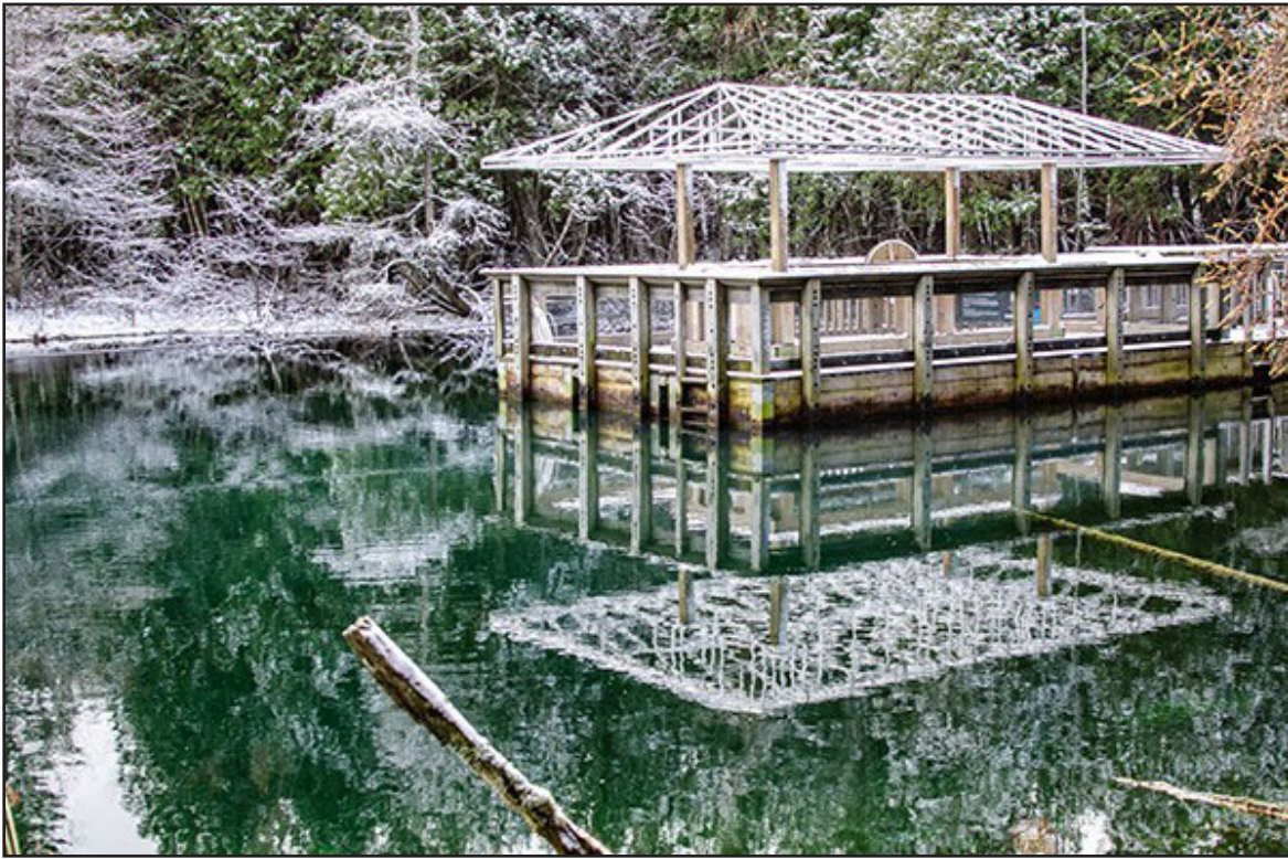
The raft at the Big Spring at Palms Book State Park in Schoolcraft County is shown on a winter day. Photo courtesy of Michigan DNR.
