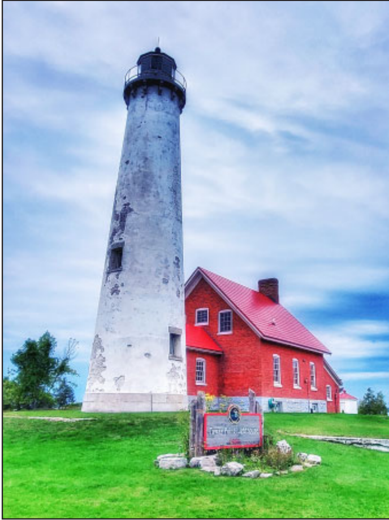
Previous restoration had covered the brick tower in a cement coating called parge. By 2020, the parge had failed along the tower, damaging original brick. Photo courtesy of Ana Eastlick, 2020 Michigan State Parks photo ambassador.
