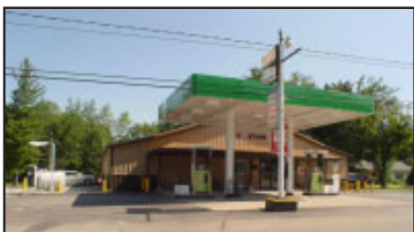
Barton City – BUY YOURSELF A JOB AND LIFESTYLE that is located in the heart of the Huron National Forest in lower northeast Michigan. This convenience store/gas station is located in Barton City. 22-0064 $499,900
