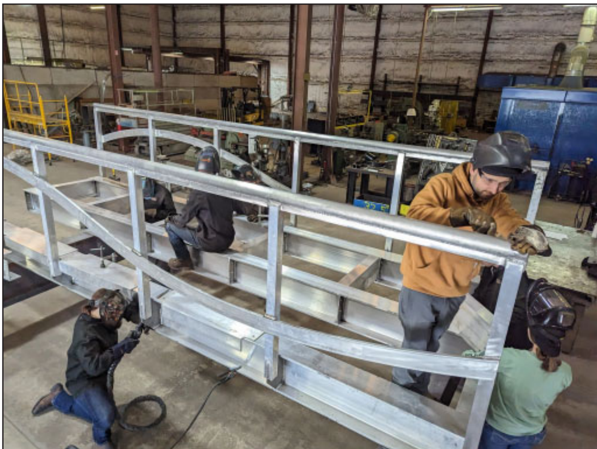
Industrial Arts Institute student welders and fabricators work on the footbridge that is expected to be installed this summer at Harrisville State Park. Photo courtesy of Michigan DNR.
