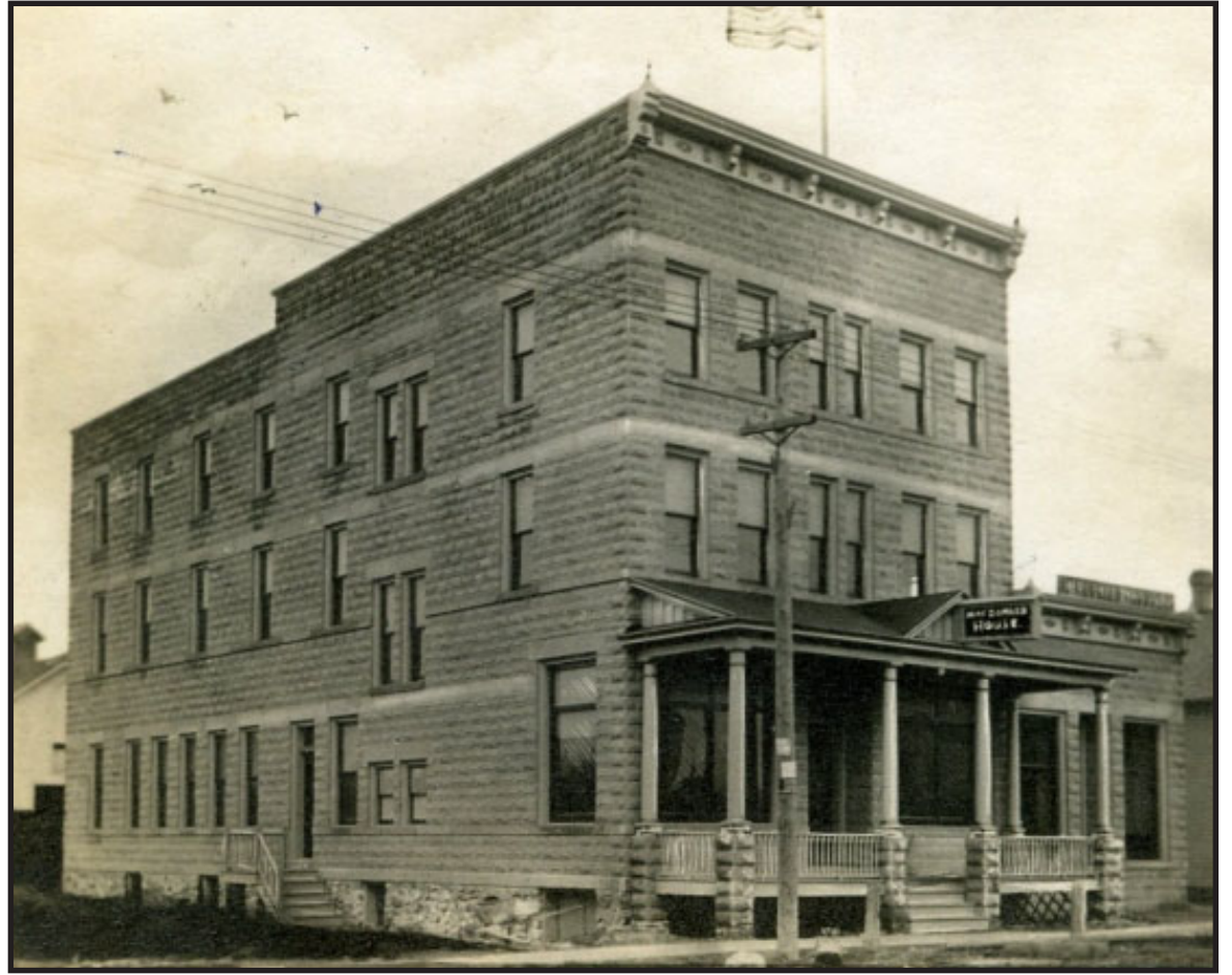
McDonald House destroyed by fire Friday, May 5, 1922. The building was one of the finest hotel structures on the Huron shore. It was built by Charles J. MacDonald and thrown open to the public the second week in April, 1907. The main building was 32x80 with three stories and the annex was 20x70, with basement under all. It was cement veneered and the interior finish was of southern pine with maple floors and steel ceilings. Steam heat, electric light, running water, baths. The dining room was 30x30, which with commodious lobby, reception room, kitchen, etc., occupied the first floor. The second and third floors were occupied by 26 guest rooms and ladies' parlor. There were no "inside" rooms, all having windows opening out of doors. The first manager of the hotel was Harry H. Purkiss and the barroom was presided over by George Emeigh, assisted by Jos. Racine. Photo from Alcona Review archives.
