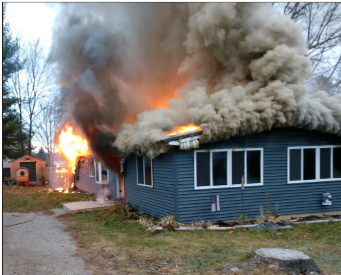
No one was inside this home on Merrick Drive in Lincoln when fire broke out Sunday morning. Courtesy photo.
