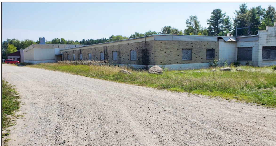
The former factory building on Third Street in Harrisville (which is just north of the Harrisville State Park property border) will see demolition to the building in the foreground (Building A) and the closure of the gravel road to pedestrian and vehicle traffic. Photo by Cheryl Peterson.
