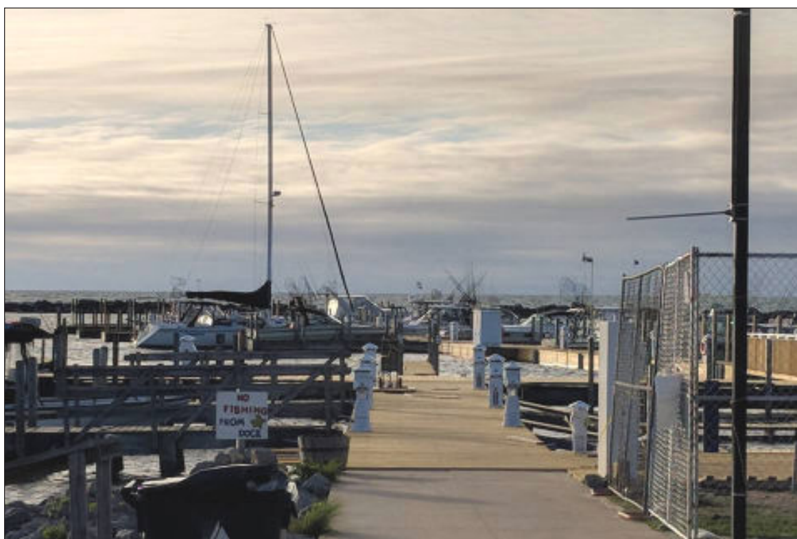
The Harrisville Harbor of Refuge is wrapping up the final stages of phase one and two of construction just in time for the summer boating season. The construction included a new main spine for the south dock; re-decking all of the fixed docks up to, but not including, the gas dock; installation of new mooring cleats for all fixed dock slips; rerouting/replacing all electrical systems on the fixed dock and south docks and bringing them up to code; replacing all water/plumbing from the shore line to all fixed docks and south dock; installation of service towers for all slips; installation of new safety stations with United States Coast Guard approved type IV life rings and fire extinguishers; and installation of a new bubbling/ice suppression system on the south floating docks, including the reused finger piers which will eventually be replaced in phase five. Courtesy Photo.
