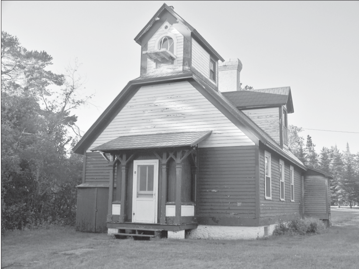
The 1868 Copper Harbor Range Lighthouse is shown prior to the start of restoration efforts, which are ongoing. Photos courtesy of Michigan DNR.
