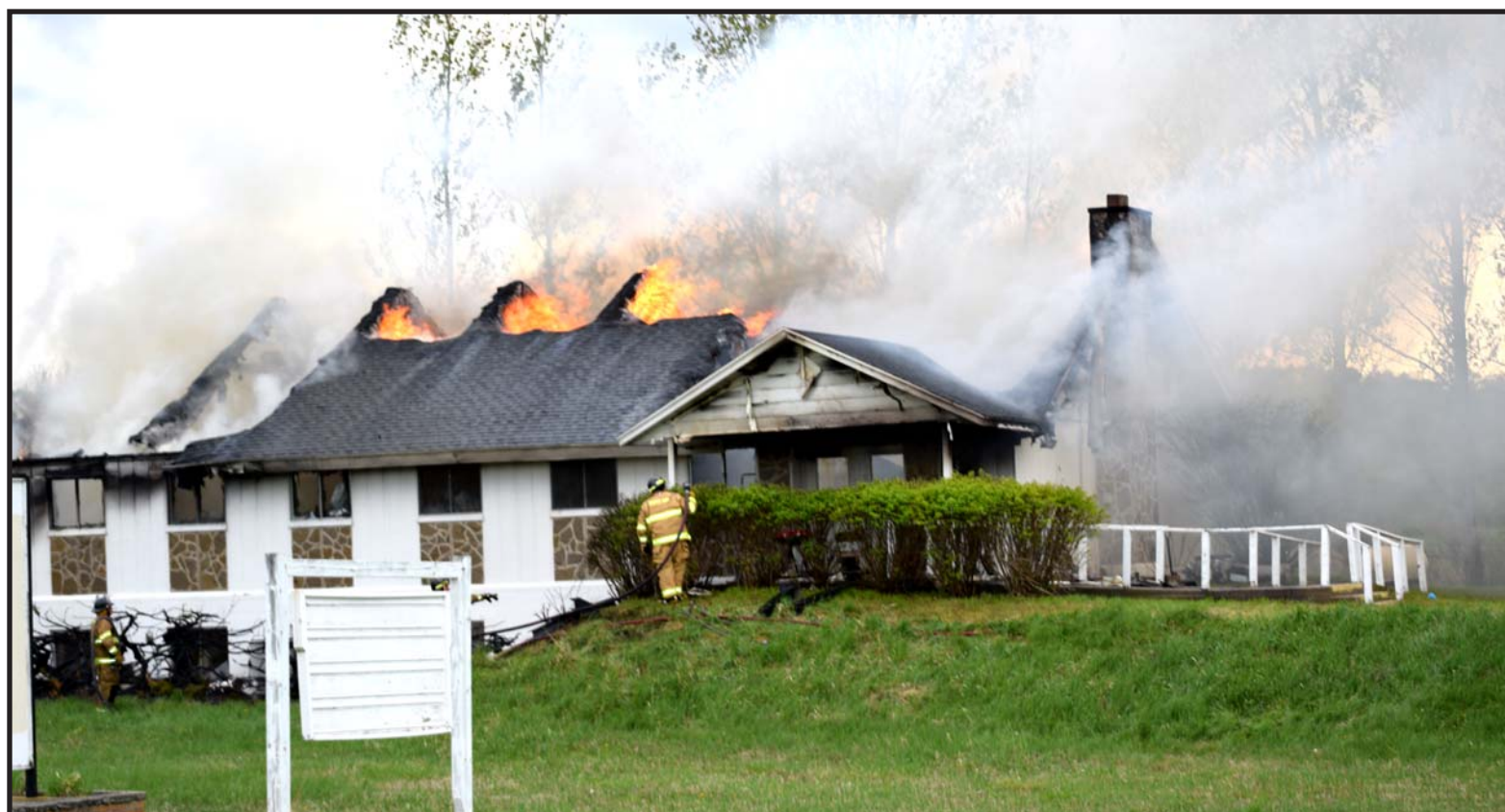
Local fire fighters from four departments spent more than five hours battling the fire that destroyed this former church in Curran. Photo by Kirk Walton.
