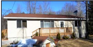
Mikado -Two bedroom, 2 bath home with sizable yard and a insulated custom shed to work on projects in. $79,900 15-0011
