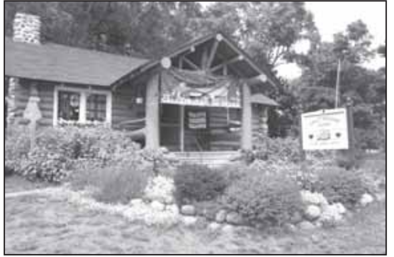
The cabin, located on the corner of US-23 and M-72 in Harrisville, was built in 1937 as a result of a public works program. A craft cooperative was formed in 1982, and the Craftmakers' Cabin was developed. Photo by Mary Weber.
