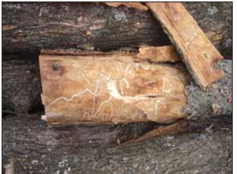
This ash tree, removed from on Monday, clearly shows the trails of emerald ash borer damage. The invasive species' larvae eat the "phloem" directly beneath the bark. The rings on the tree indicated it was more than 50 years old. Photo by Art Kniep.
