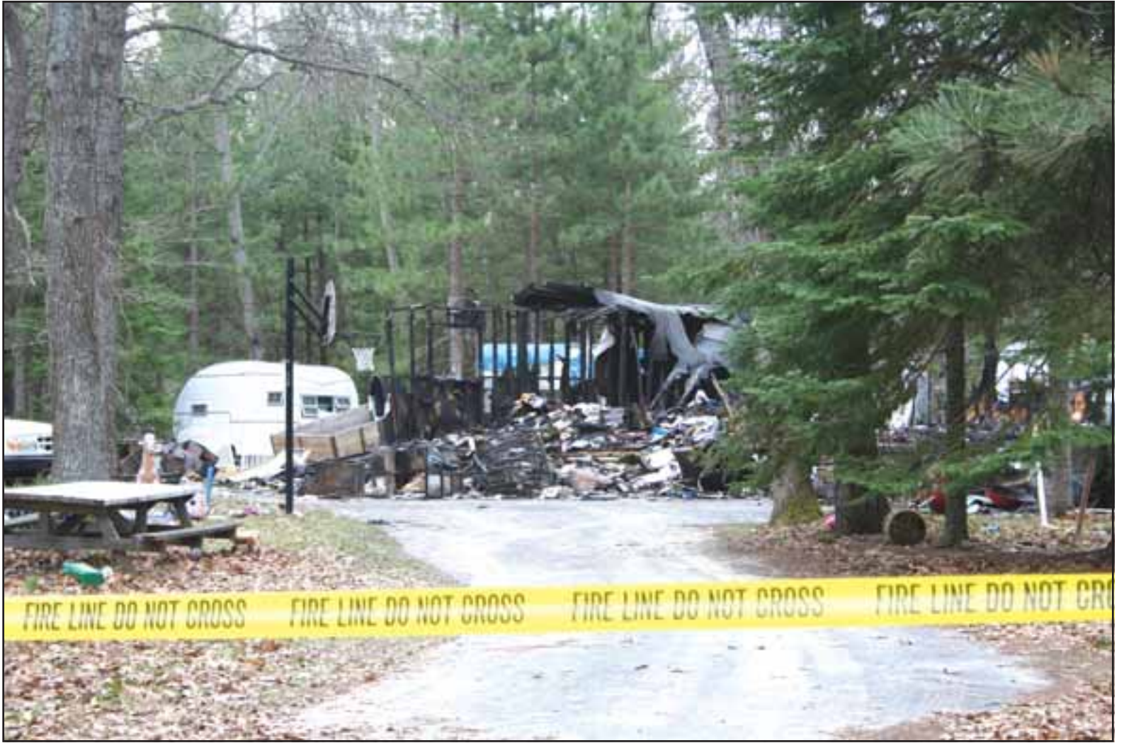
The scene of the fire (above) on Kahn Road in Mikado is still under police jurisdiction as investigators work to determine the cause. Photo by Cheryl Peterson.
